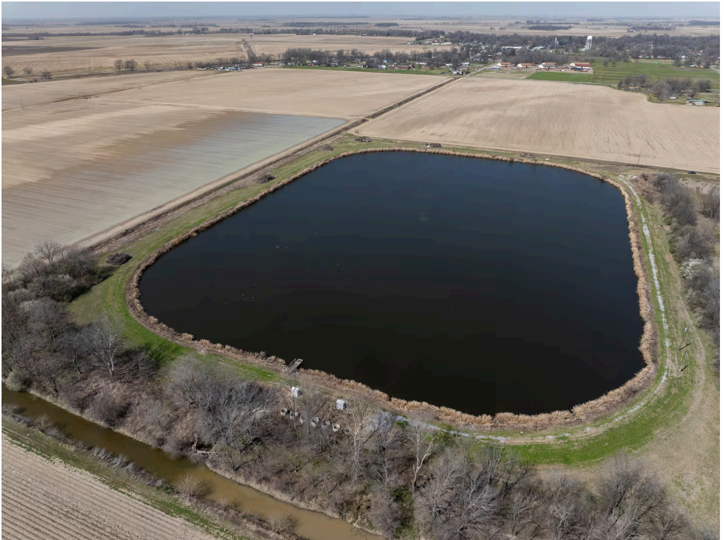
Sewage pumps throughout Shaw pump wastewater away from town, to a wastewater treatment lagoon on its outskirts. When heavy rains overwhelm the pumps, sewage pipes and drains overflow. RORY DOYLE FOR THE BOSTON GLOBE
